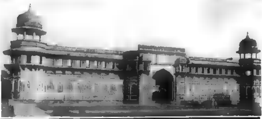
Fig. 5. Agra Fort, "Dībhāngī Mahall", exterior, land front. (Photo P. A. Andrews)
